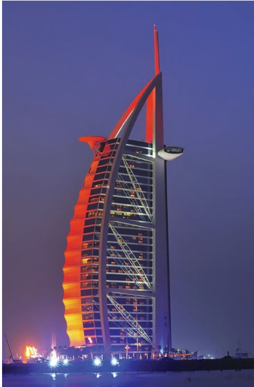
Figure 3.10 Dubai's Burj Al Arab is favorably positioned along many determinant attributes like personal service, level of physical extravagance and location
